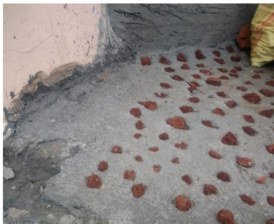
Figure 4: Brick bat coba
