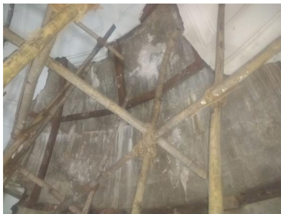
Figure 2:POP sheets and battens removal
