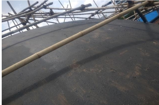
Figure 1:Dome external surface with lime mortar
